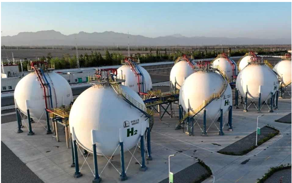
출처: Sinopec, Hydrogen storage tanks at Sinopec's 260MW Kuqa green hydrogen project
